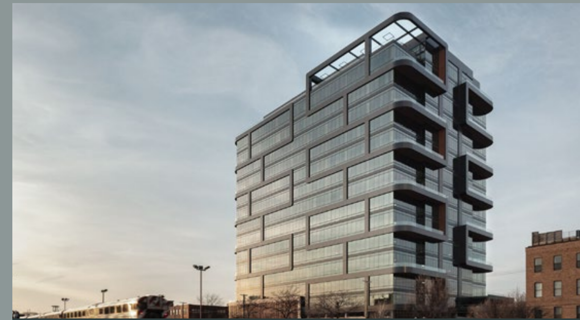
400 N Aberdeen (Delivered 2022)
